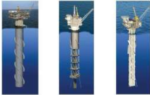
Fig. 1: Types of Spar (a) Classic Spar, (b) Truss Spar, (c) Cell Spar
